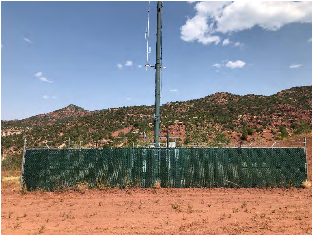
Site Photograph 3 – Looking northeast at the Subject Property.
